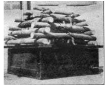
An indoor "campfire." the top base is hinged, and the box contains bulbs, incense pans, fan, etc. Note connection plug at corner.
