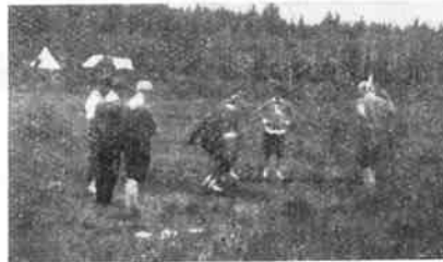
LAYING a track problem at the Nova Scotia Gillwell.
