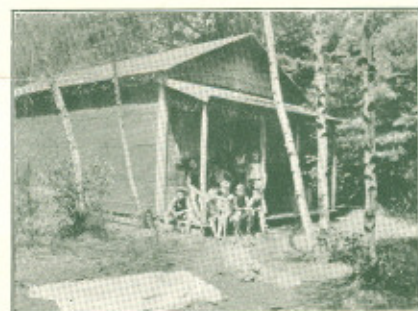
THE summer home of the Amherst Troop, Montreal,—a 25-ft.-square bunkhouse (built by the Troop). There are three bunk tiers on each side, 24 in all, with room in each for two boys; and 25 x 16 of clear floor.
