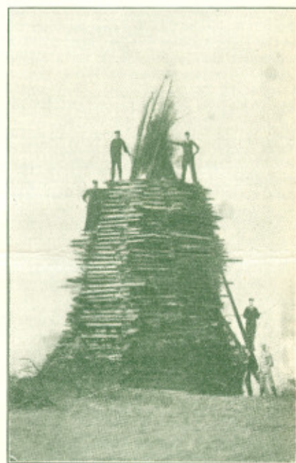
A GOOD type of large beacon of maximum duration—a 30-foot hexagonal pyramid. Lighted at the top, it burns downward, like a torch, and collapses inward.
