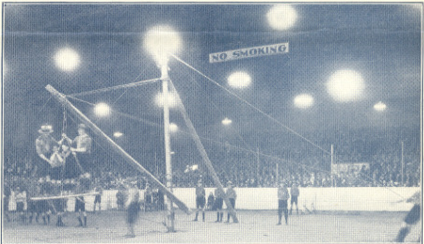
THE boom derrick run up by the Rockyford Rovers at the Calgary Baden-Powell rally. It proved itself by lifting two Rovers and a pair of Wolf Cubs.
