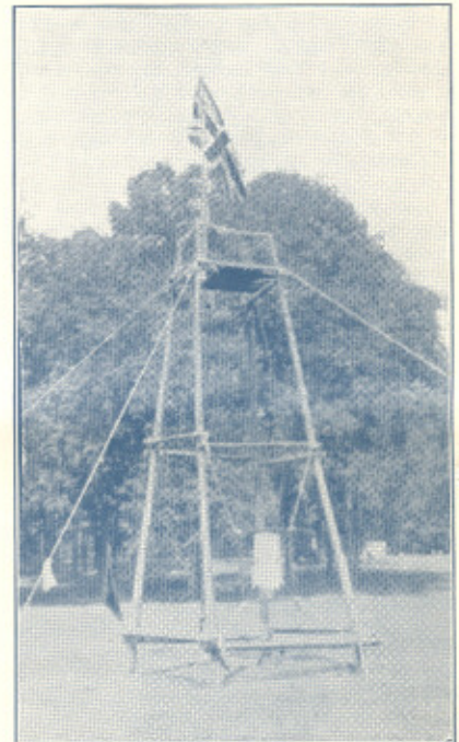
IN a more conventional setting the 10th Brantford Troop, Ont., got their signalling romance by building a tower that topped the surrounding trees.
