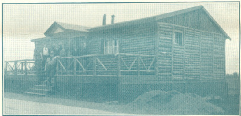
"Believe it or not,"—the end of two old freight cars, and possibly the finest Rover den in eastern Canada. The home, and the work, of the 1st St. Johns, Que., Kenneth Murray Crew. (See story on opposite page.)
