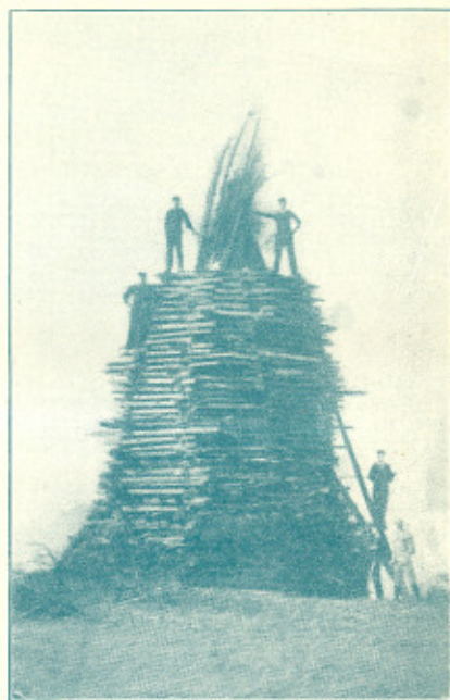
A good type of large beacon—a thirty-foot hexagonal pyramid. Lighted at the top, it burns downward, like a torch, and gradually collapses inward.
