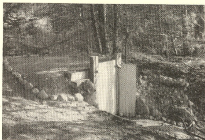
3RD HALIFAX TROOP'S CAMP ICE BOX AT GLEN HAVEN N.S. THIS BOX, BUILT INTO THE SIDE OF A BANK USED ONLY ONE PIECE OF ICE EVERY THREE OR FOUR DAYS. READ DESCRIPTION IN JUNE LEADER.
