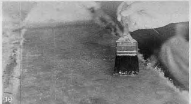
10 We applied another coat of resin to the top and bottom to get a smoother surface.
