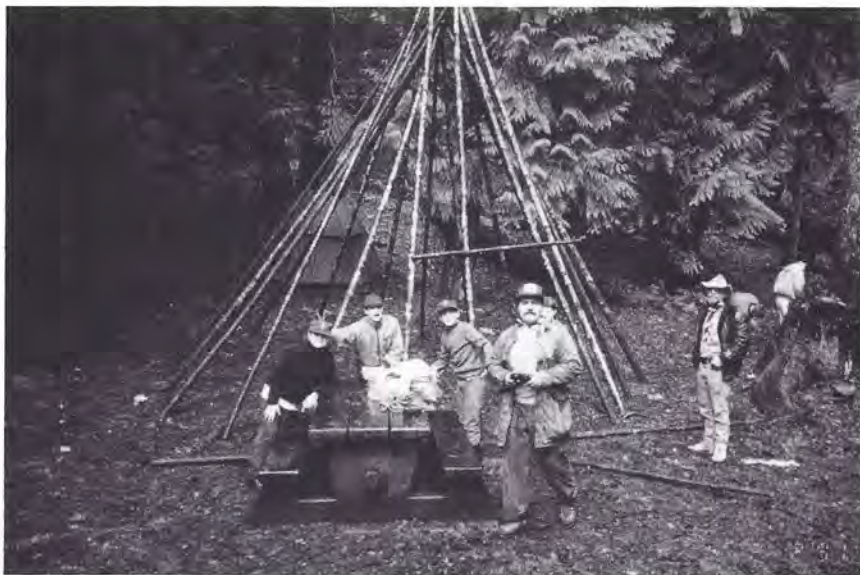
The pole frame takes shape.
