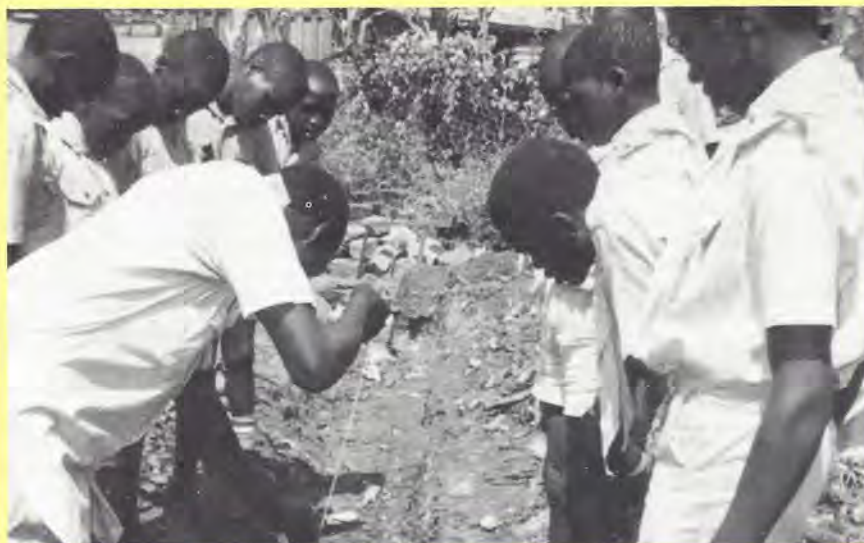
A technical expert shows Bwaise Scouts how to level the foundation before laying handmade bricks to build a chicken house in Kampala District, Uganda. The poultry project, sponsored by the Blue Water Region, Ont., gave groups like the 4th Goderich some fun, too, says Mary Anne Rowlands, field executive. During the promotional meeting, live chickens paid a visit and Goderich Beavers decorated the walls with their posters of chickens and chicken farming. The Egg Marketing Board let the group use "Let's Get Cracking!" materials for fundraising and, each time an egg was cracked in a member's home during March, 10 cents was put aside for the poultry project. Mary Ann says the 4th Goderich raised almost $800 for Uganda.
