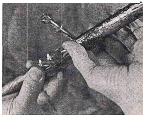
2. PLACE THE REPAIR clamp around the pipe and pinch it closed. Slip the bolt between the two iron prongs.
