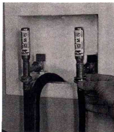
2 CONNECT THE hoses to the ends of the arresters. If the hoses are cracked or brittle, replace them.
