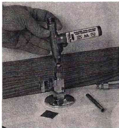
2 ATTACH THE arrester to the short stub of tubing protruding from the toilet's shutoff valve.
