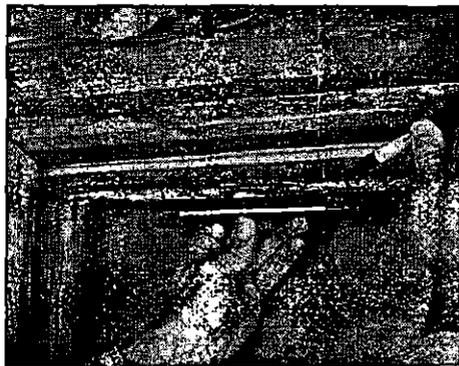
**1** 1. HOLD the compression repair coupling against the damaged pipe and mark 1 in. in from each end.
