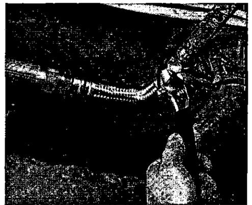
**5** 5. USE TWO WRENCHES to install the flexible connector. Hold the connector nut stationary and turn the compression nut.
