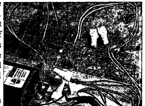
**CONNECT THE LEADS from the new ballast to the fixture wiring with wire nuts. Tighten them firmly.**
