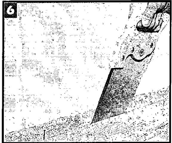
**6** Internal stresses in wood can cause it to bind on long rips. Insert a nail in the saw kerf to open space for blade.
