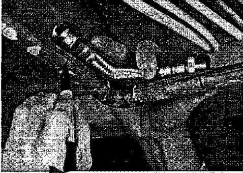
**1** 1. HOLD the Quick-Fix connector against the leaky elbow fitting, then mark where the pipes need to be cut.
