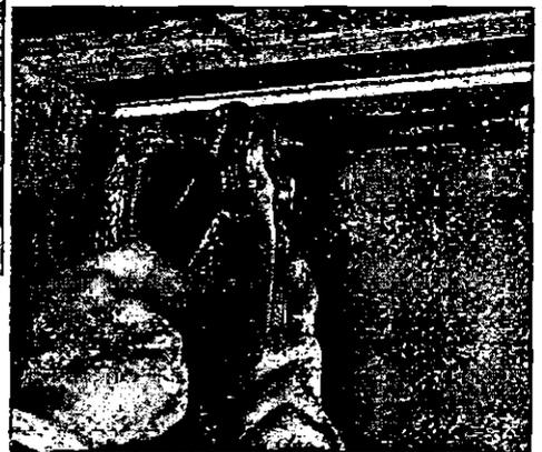
**4** 4. HOLD the nut on the coupling with one wrench and use a second wrench to tighten the compression nut.
