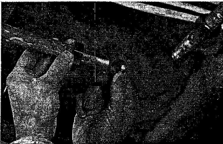
**4** 4. SLIP THE COMPRESSION nut over the pipe end, then slide on the ferrule, also called the compression ring.
