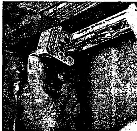
**2** 2. WHEN space is limited, use a miniature tubing cutter to cleanly slice through the copper water pipe.
