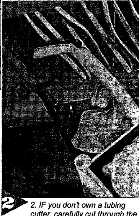
**2** 2. IF you don't own a tubing cutter, carefully cut through the copper pipe with a hacksaw or reciprocating saw.
