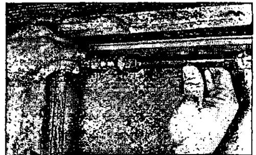
**3** 3. SLIP the repair coupling into place after sliding the compression nuts and ferrules onto the ends of the pipe.
