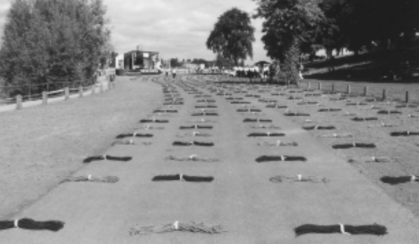
The rope layed out ready to start.
