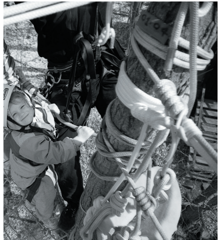
Two modified Tarbuck knots securing safety lines, Kilcoo Camp Aerial Course, Minden, Ontario, Canada; Photo: Hai Pham. Note that the two safety lines are seized together to facilitate ease of clipping carabiners.
