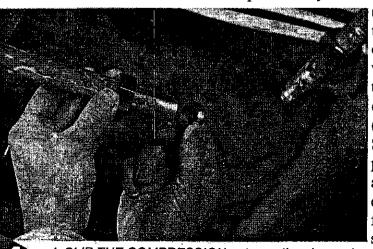
4. SLIP THE COMPRESSION nut over the pipe end, then slide on the ferrule, also called the compression ring.
