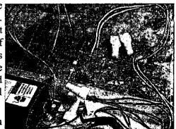
CONNECT THE LEADS from new ballast to the fixture wiring with wire nuts. Tighten them firmly.
