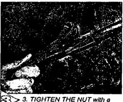
3. TIGHTEN THE NUT with a wrench to compress the thick rubber gasket and plug up the pinhole-size leak.
