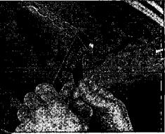
3. BUFF THE JUST-CUT pipe ends with a strip of emery cloth. Be sure to remove all burrs and rough spots.
