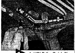
1. HOLD the Quick-Fix connector against the leaky elbow fitting, then mark where the pipes need to be cut.
