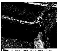
5. USE TWO WRENCHES to install the flexible connector. Hold the connector nut stationary and turn the compression nut.
