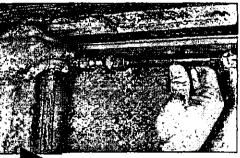
. 3. SLIP the repair coupling into place after sliding the compression nuts and ferrules onto the ends of the pipe.
