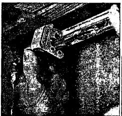
2. WHEN space is limited, use a miniature tubing cutter to cleanly slice through the copper water pipe.
