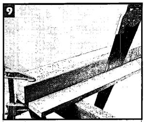
For straight rips, guide ripsaw with a length of 2 x 3 stock. Align guide with cutline and clamp in place.
