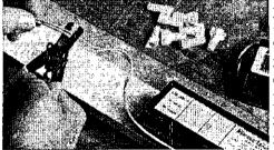
AFTER CUTTING the power or unplugging the fixture, remove the old one to an electrical-supply house. access panel and clip the leads from the old ballast.
