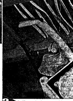
\* 2. IF you don't own a tubing cutter, carefully cut through the copper pipe with a hacksaw or reciprocating saw.
