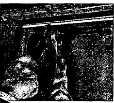
4. HOLD the nut on the coupling with one wrench and use a second wrench to tighten the compression nut.
