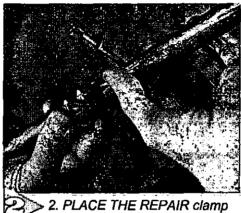
2. PLACE THE REPAIR clamp around the pipe and pinch it closed. Slip the bolt between the two iron prongs.
