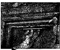
■ 1. HOLD the compression repair coupling against the damaged pipe and mark 1 in. in from each end.
