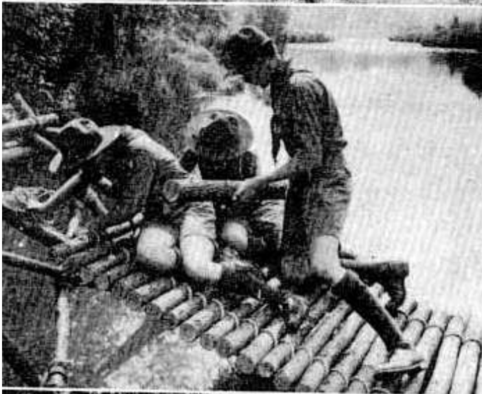
Middle: Finishing the floor. The first bottom floor piece was square-lashed to the ramp timber.
