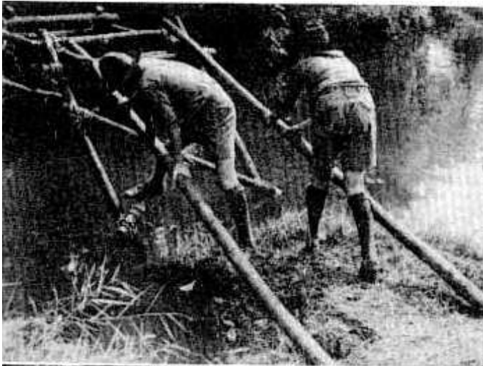
Top: Placing the ramp timbers. Length depends on shore line.
