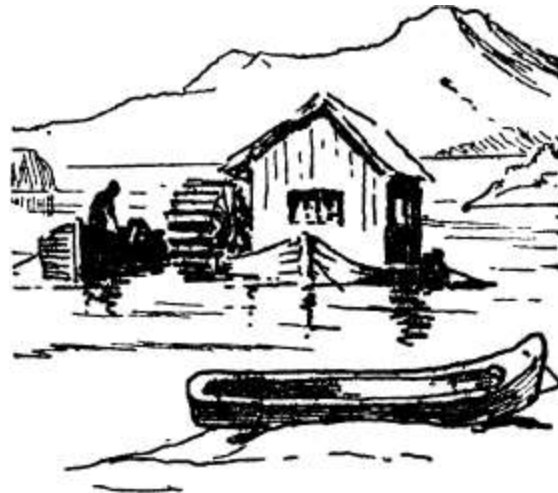
WATER-MILLS IN BOSNIA ARE ERECTED ON BARGES ANCHORED IN THE MIDDLE OF THE STREAM
